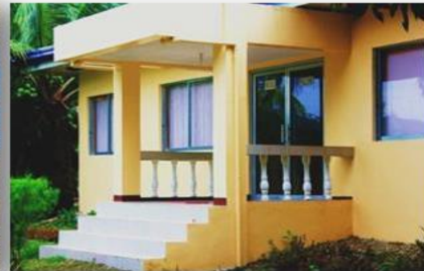
Mess Hall/ Processing Unit
