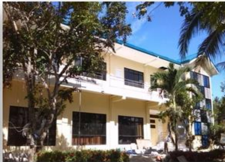
Multi Purpose Building & Dormitories
