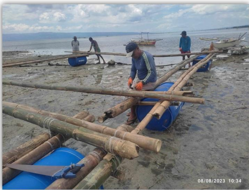
Construction of Bamboo Frame and Net Cages at Bais City
